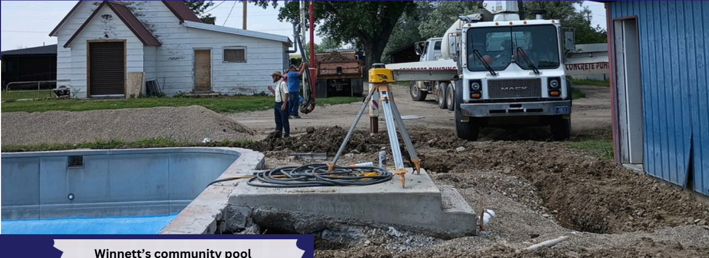
Winnett's community pool getting its new deck poured!
